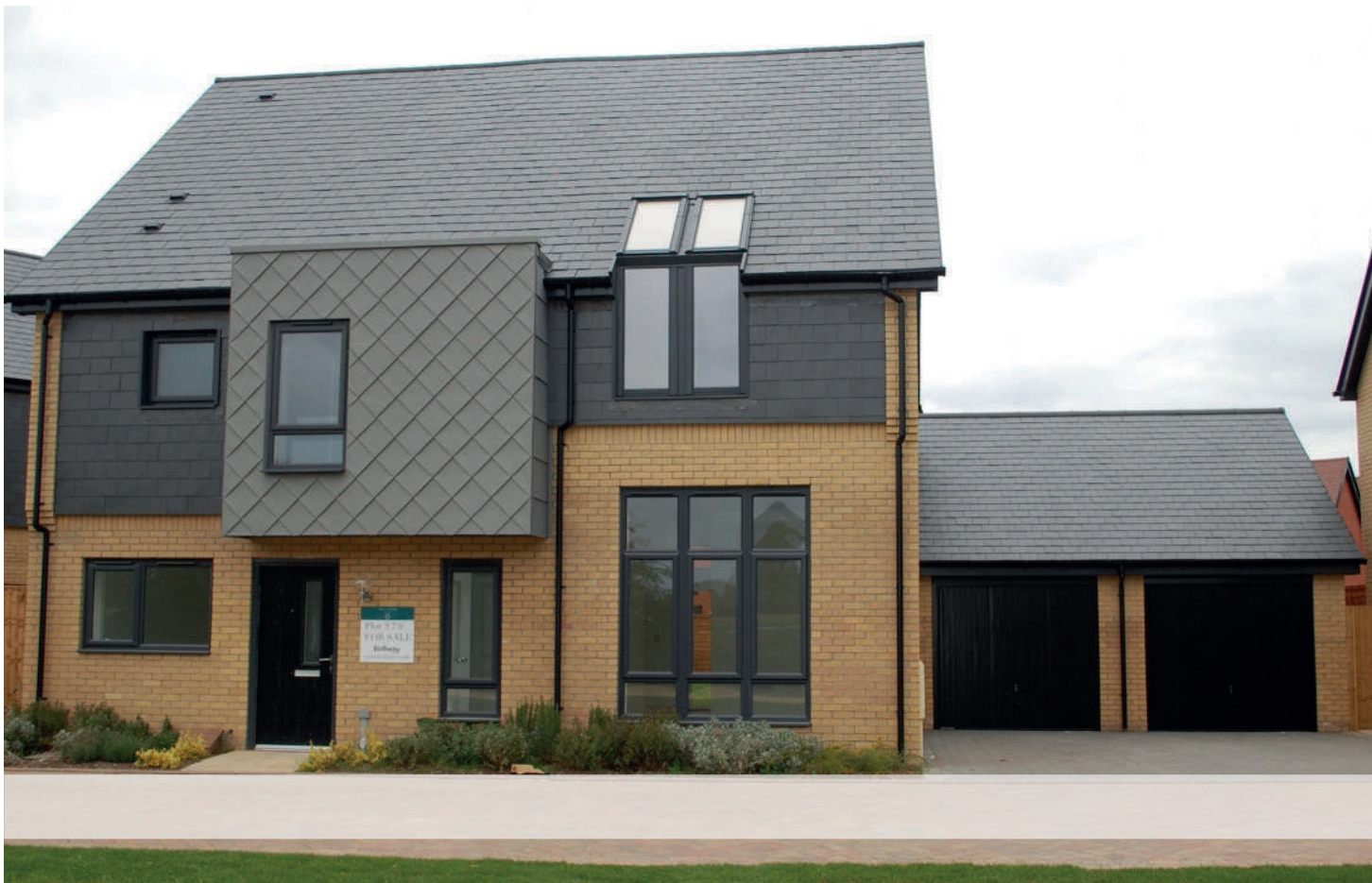
Classic First Mix Grade. Bellway Homes, Chelmsford, Essex.
